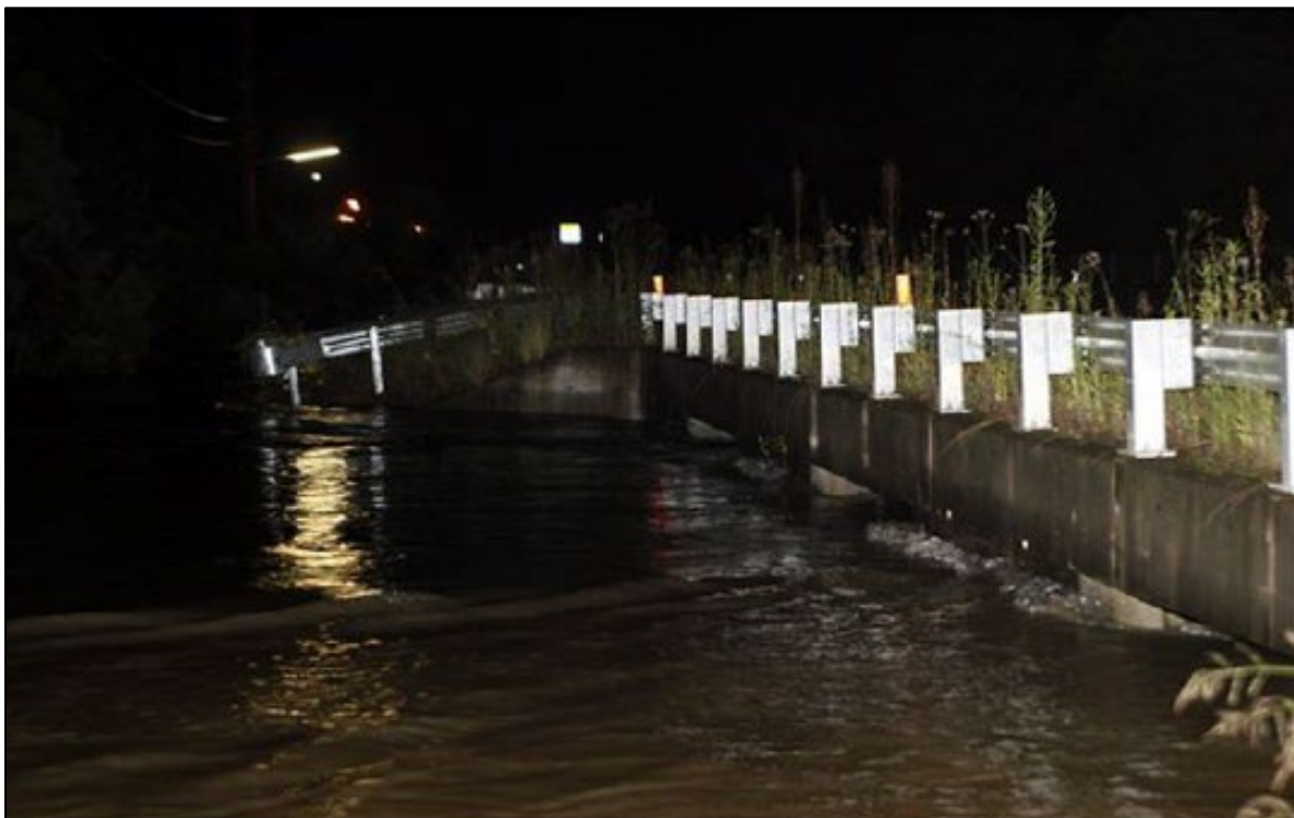
Plate 1 Photo of Londonderry Road culvert captured on 9 February 2012
