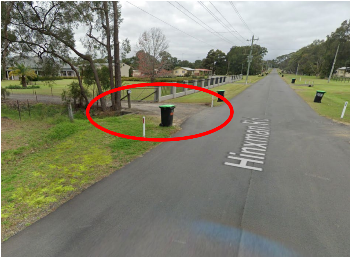
Plate 28 Location of built up ground near the upstream end of the drainages wale. Photo courtesy of Google Streetview ©
