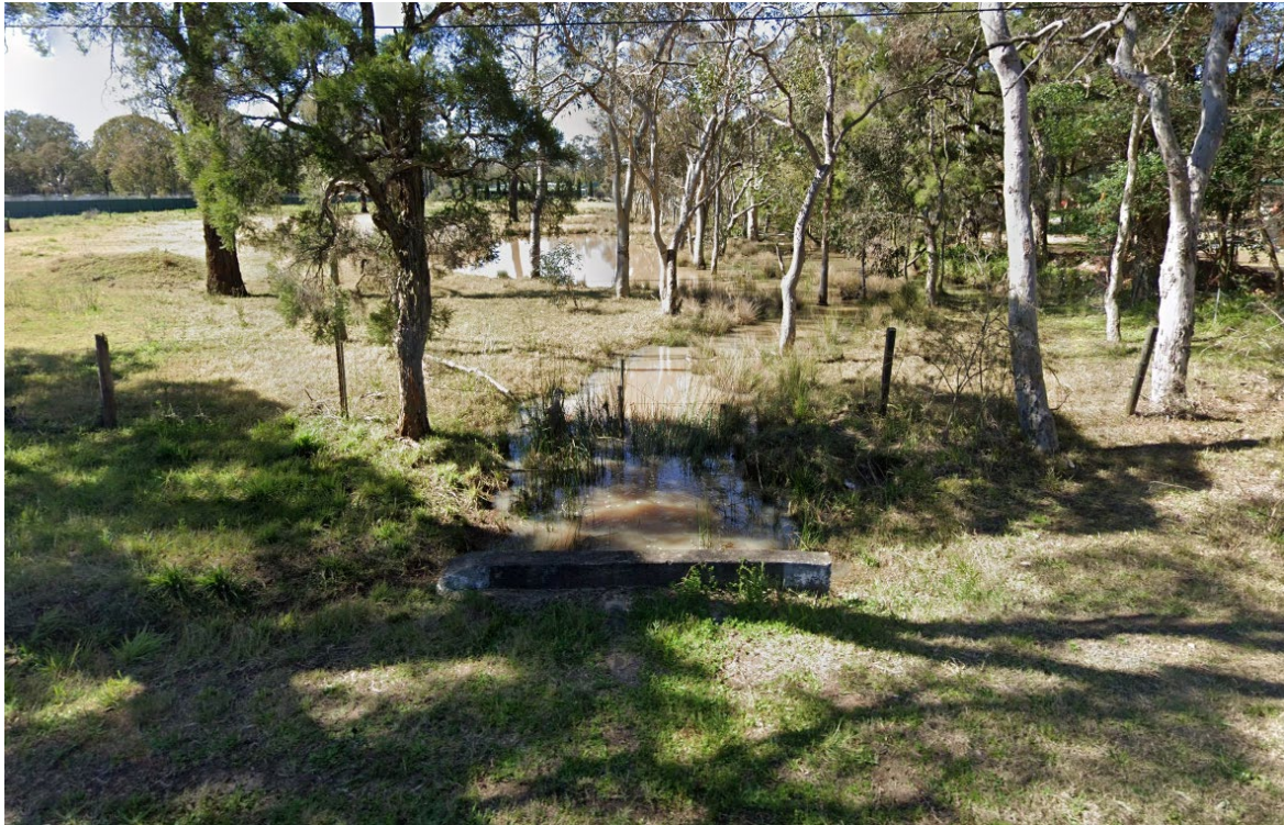
Plate 25 Torkington Creek channel at Nutt Road (looking east). Photo courtesy of Google Streetview©
